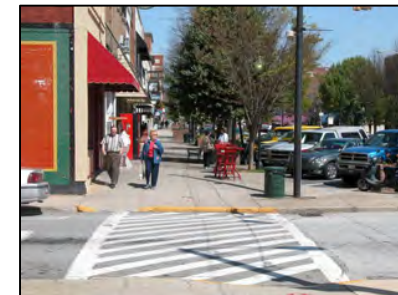
Example of high visibility crosswalk not aligned with curb ramp
