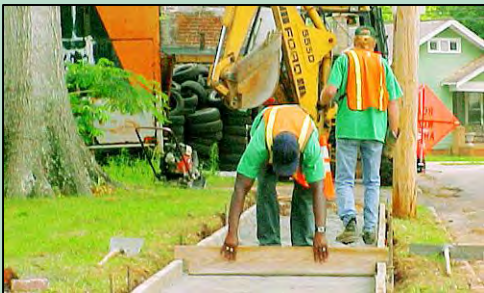
Example of sidewalk construction
